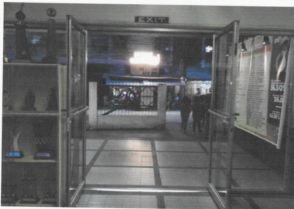
EXIT WITH SIGNAGE AT COLLEGE OF ENGINEERING AND ARCHITECTURE BUILDING
